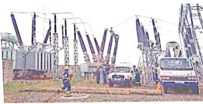
Kenya Power workers at the Embakasi Sub-station ahead of the commissioning of an underground cable at the National Park last May. The project is part of the Nairobi Ring project.
