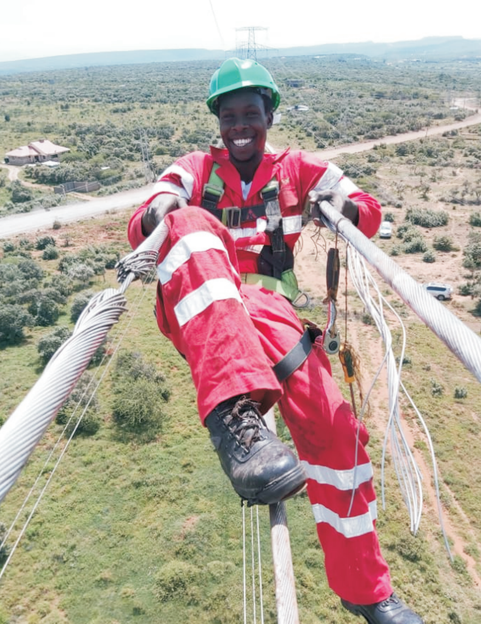
KETRACO O & M Team patrol transmission lines to identify faults and undertake remedial work to avert breakdown. Craftman Johnson Kapsowe (Above) poses for a photo atop 400 kV Suswa - Isinya TL during maintenance works on the line.
