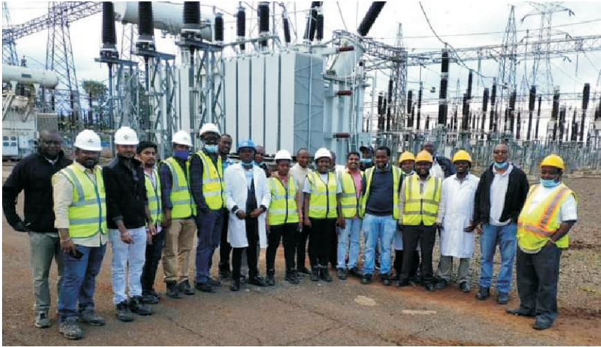
Nairobi North substation, part of the System Reinforcement Component of Eastern Electricity Highway Project, has an improved capacity after a 90MVA transformer T6 was added and energised.
