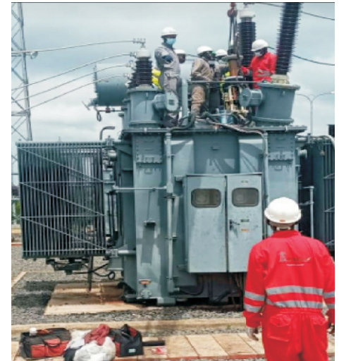
Transformer Maintenance work ongoing at Rang'ala Substation. The company attaches a lot of seriousness on maintenance works on her transmission line projects.
