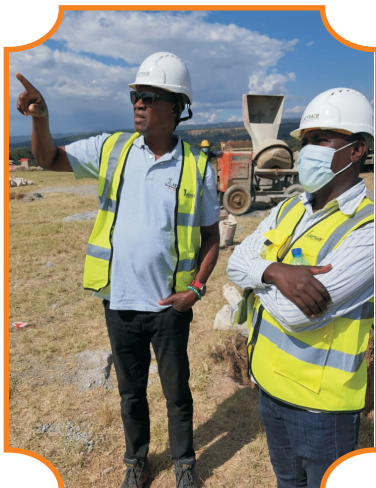
Chairman of KETRACO Board of Directors Hon. Eng. James Rege, CBS in discussions with OLK's resident engineer James Kairu regarding the status of the ongoing construction works during a Board inspections tour.
