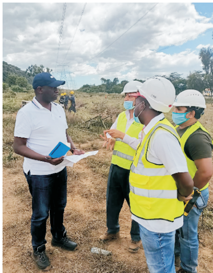
Energy CS Hon. Charles Keter, EGH when he carried out inspection on the ongoing stringing works on Olkaria - Lessos - Kisumu line at Naivasha area. The project is scheduled for completion end of January 2021.
