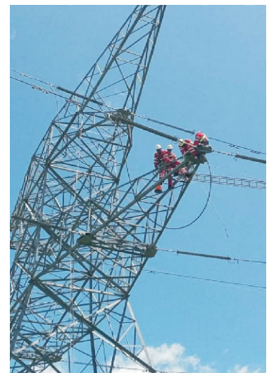
KETRACO O&M engineers at work.
