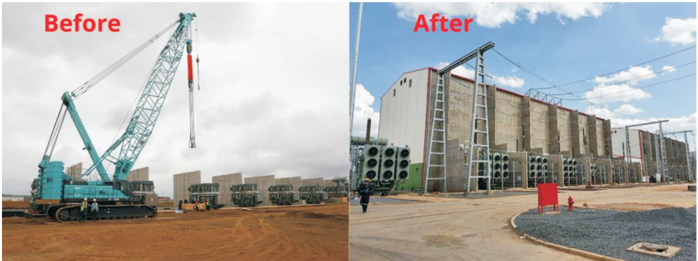
“Suswa High Voltage Direct Current (HVDC) Converter station is in the final stages of construction at 99% complete. The converter station is a component of the 1045Km 500KV HVDC Ethiopia - Kenya transmission line which is also in its final stages of construction at 98% .”
