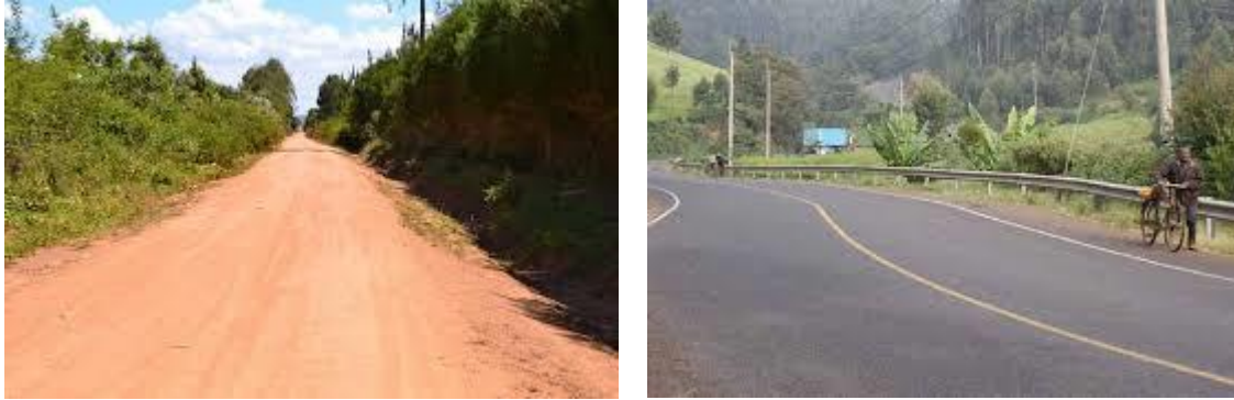
Figure 5-54: Sample of road Network within Laikipia East Subcounty Source: EMC Consultants Field Survey, 2019
