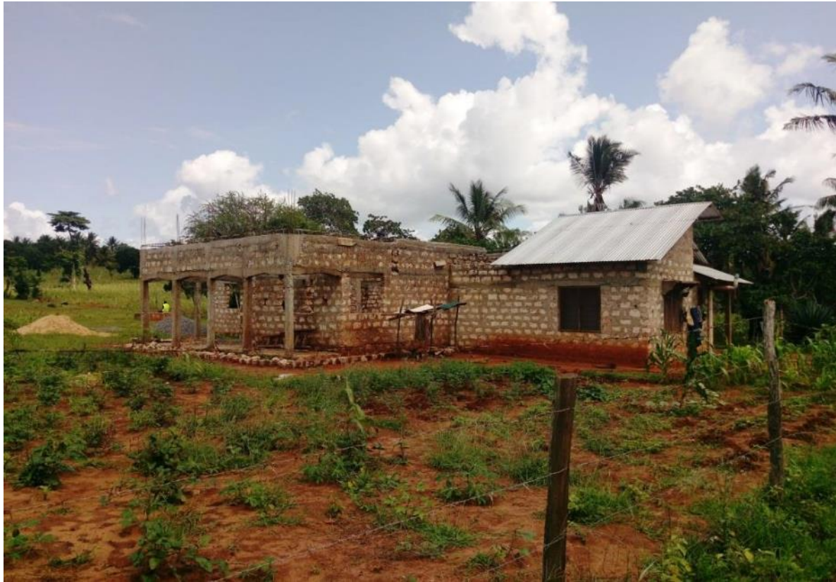
Plate 2-4 Permanent house structure along the Row Source - AWEMAC field Survey
