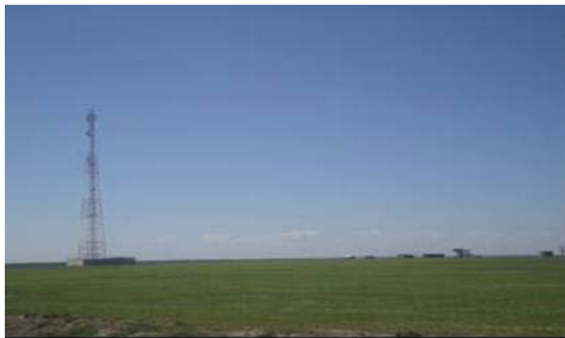
Base station along Nanyuki-Rumuruti
