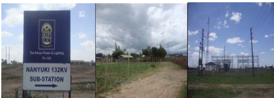
Picture 22: Existing Nanyuki Sub-station and the encroached way leave of the 132KV line from Lanet to Nanyuki (proposed for a double circuit)
