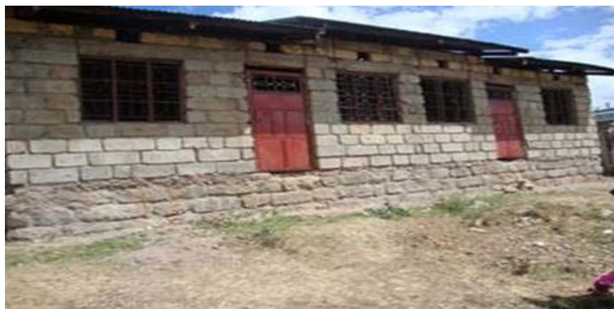
House to be affected by the transmission line
