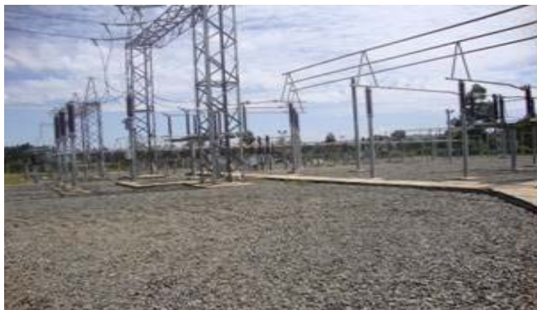
Main Grid in Lessos
