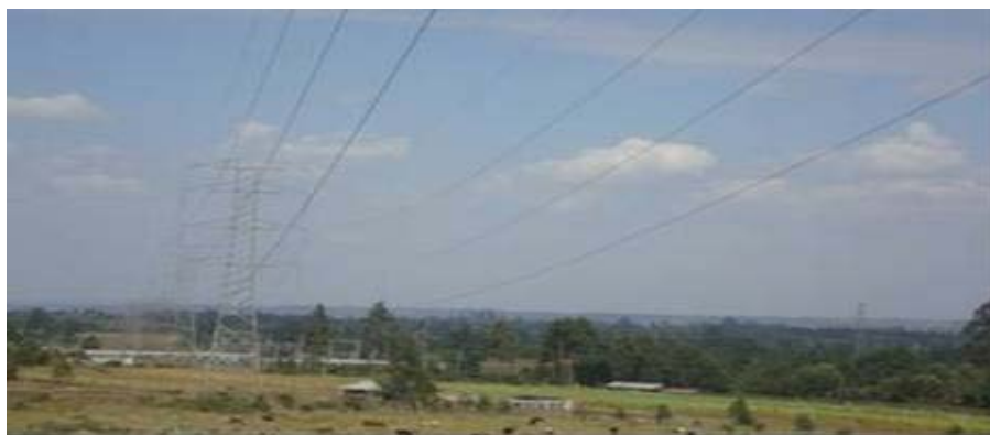
Existing 220KV Turkwel to Lessos
