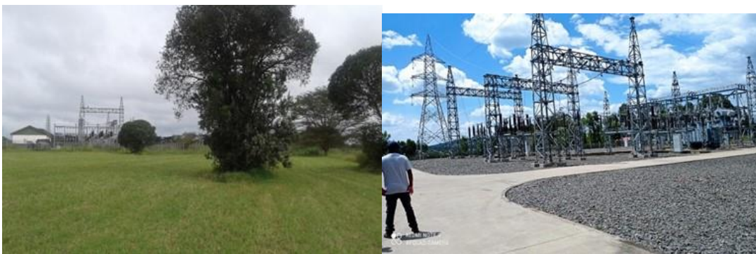
Plate 2-2: Narok 132kV substation take-off point & Bomet 132Kv substation terminal point
