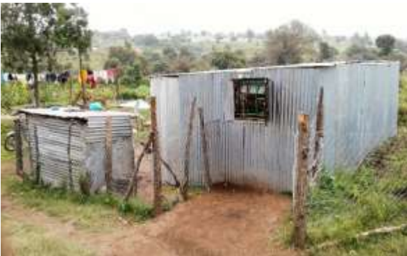
Iron sheet structure
