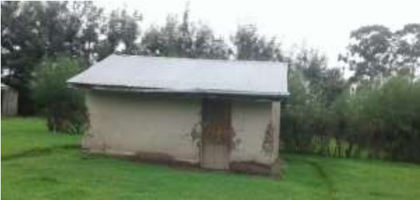
Mud walled and iron sheet roof and earthen floor
