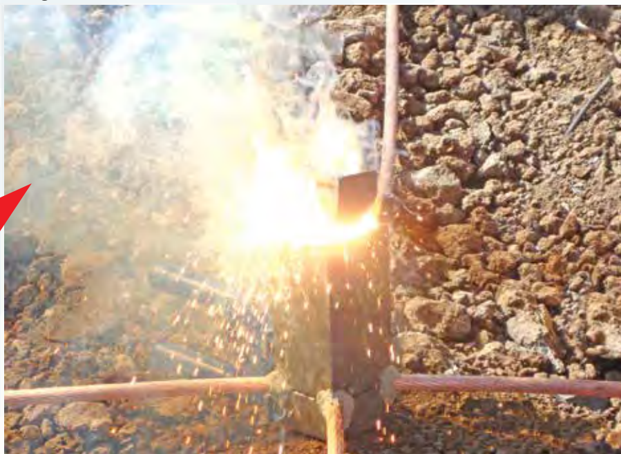
Welding Earthing Grid Isiolo Sub-station
