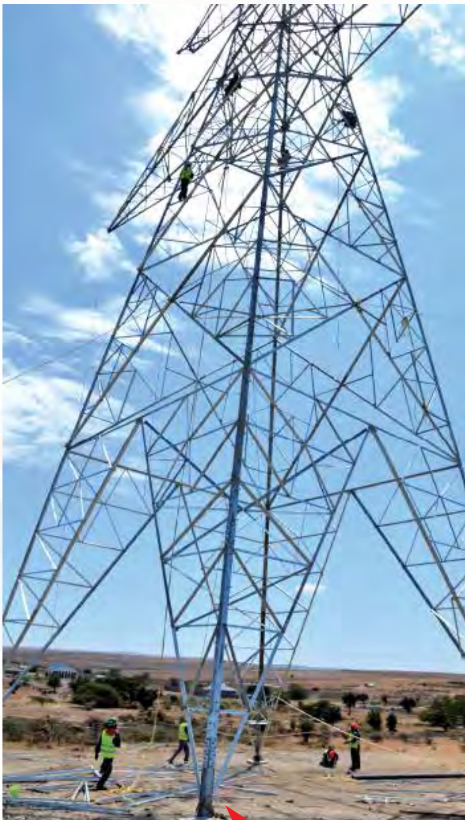
Tower erection along Suswa-Isinya line
