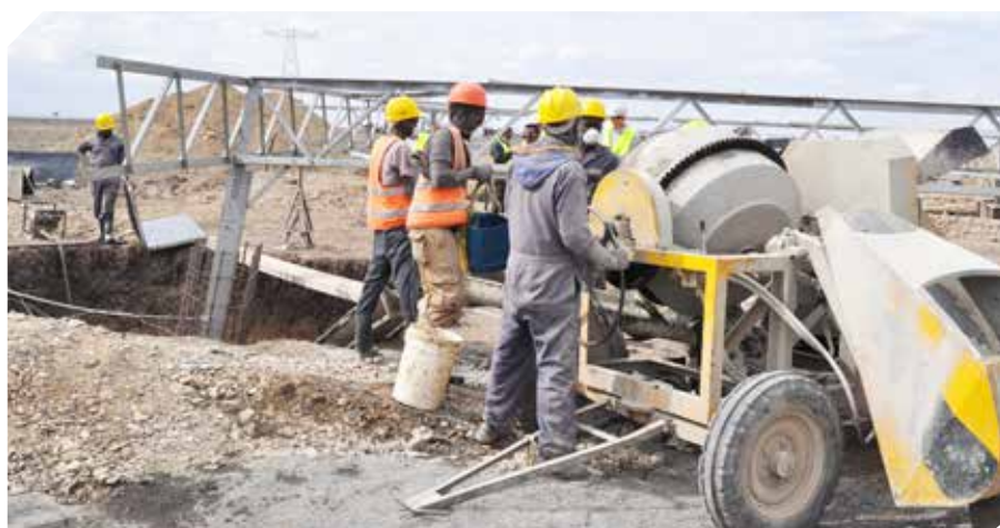
Concreting of a tower foundation along the 500kV Eastern Electricity Highway Project
