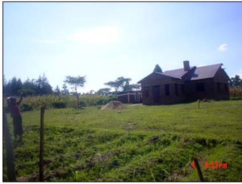
Plate1: Building Structure located between point B-C
