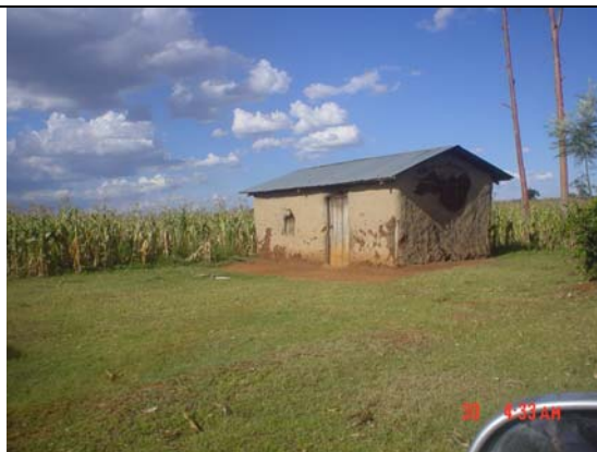
Plate 6: Lone standing housing structure on 100 acres of land in Soy near point H
