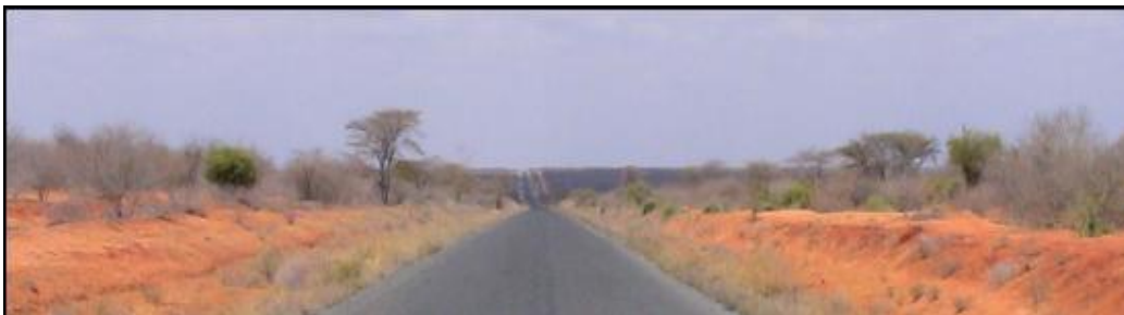
Picture 4: Typical view along the eastern section.
