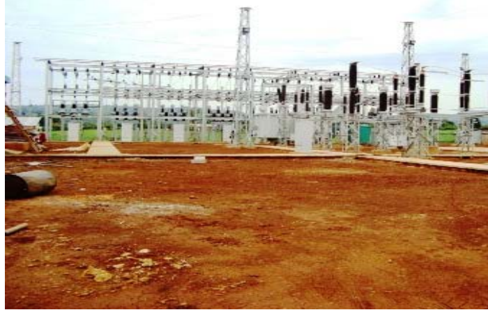
Fig.4.2: Kegati Substation under construction
