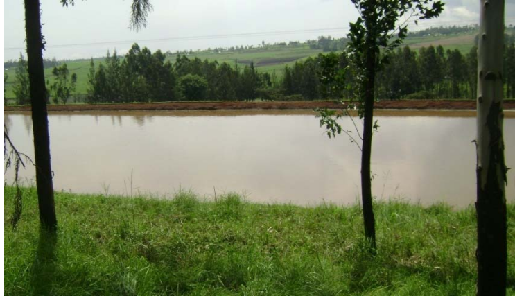
Plate 4: Sony Sugar Sewerage Treatment Plant.
