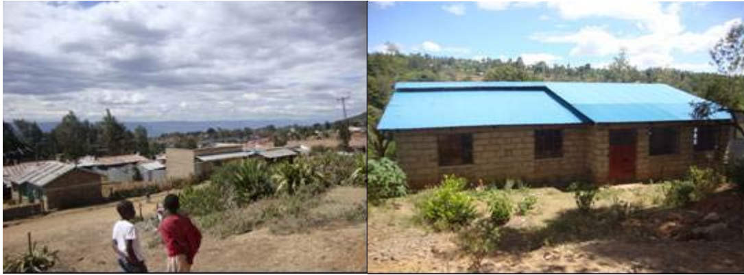
Plate 4: Permanent rental houses within Kaprogonya, Kabarnet town
