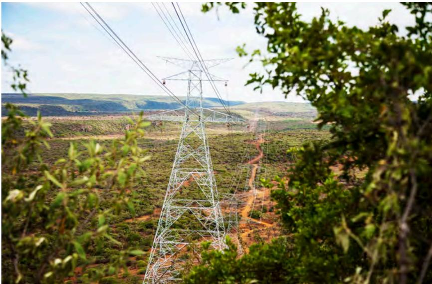
The Suswa – Isinya transmission line's special tower (6B/1). This tower is 94m high (10 m higher than Nyayo House) making it the tallest in Kenya.
