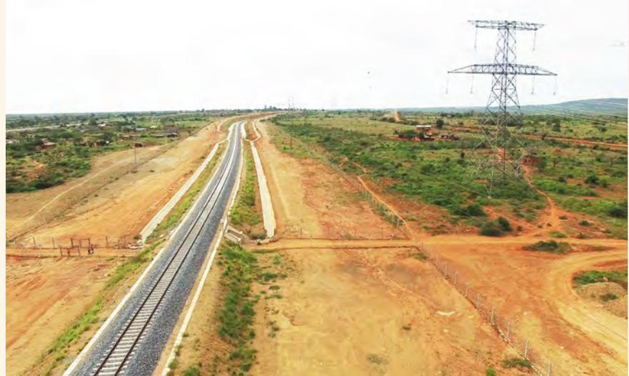
A section of the 482km 400kV Mombasa-Nairobi transmission line running parallel to the Standard Gauge Railway (SGR)
